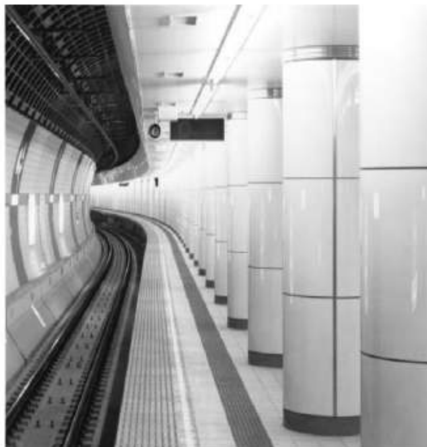
Figure 4.67 Neopariés™ glass-ceramic as a building material.
